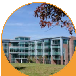
COMMUNITY BUILDING CENTRO COMUNITARIO
