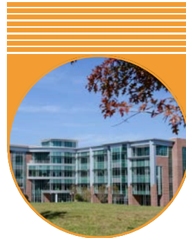
COMMUNITY BUILDING CENTRO COMUNITARIO
