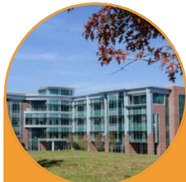
COMMUNITY BUILDING CENTRO COMUNITARIO
