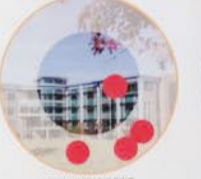
COMMUNITY BUILDING CENTRO COMUNITARIO
